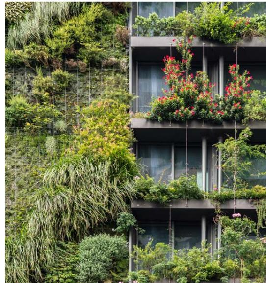
Green facades improve the air quality, produce oxygen, and filter dust, pollutants, and noise. They also provide protection against heat and cold.
