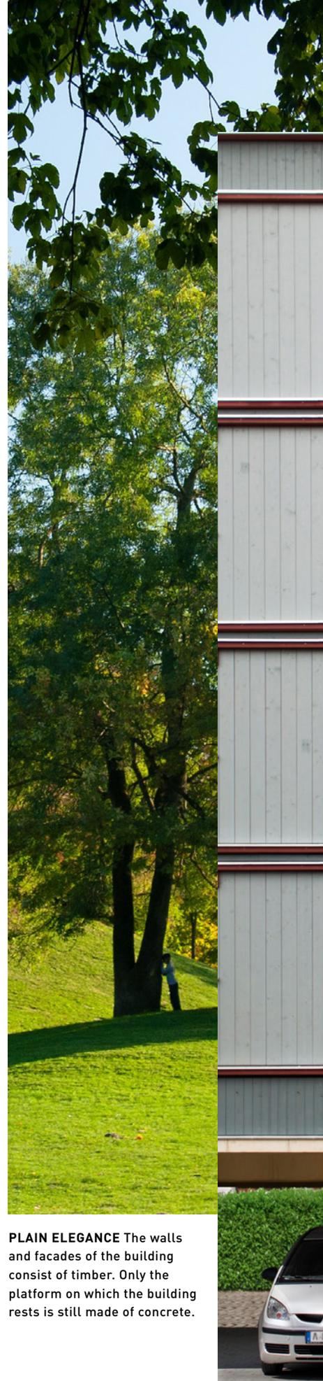
**PLAIN ELEGANCE** The walls and facades of the building consist of timber. Only the platform on which the building rests is still made of concrete.
