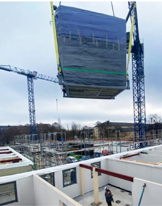
In prefabricated timber construction, cranes lift the assembled components into place within minutes. Even complete bathrooms can thus be installed into the building.
