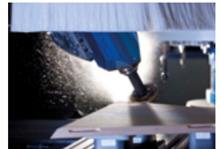
Trimming of inclined grooves for panel connection
